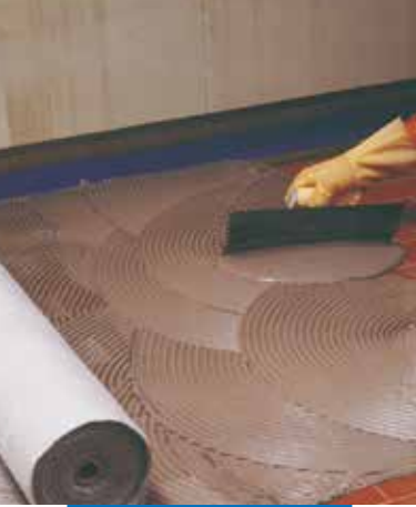
Application of the first layer of Mapelastic, and successive laying of Mapetex Sel
