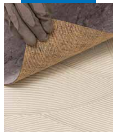
Installation of Linoleum with Ultrabond Eco V4 Evolution
