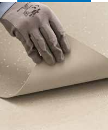
Installation of RUBBER with Ultrabond Eco V4 Evolution
