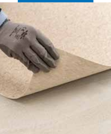
Installation of homogeneous PVC with Ultrabond Eco V4 Evolution
